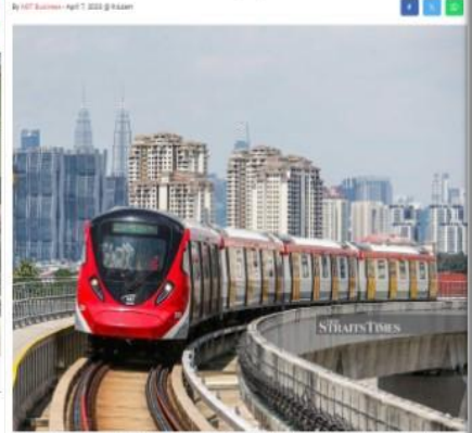
The government will likely complete the cost review of the Mass Rapid Transit Line 3 (MRT3) project by June and award construction contracts soon after, analysts say. - NSTP/ADAWATI ALIAS
